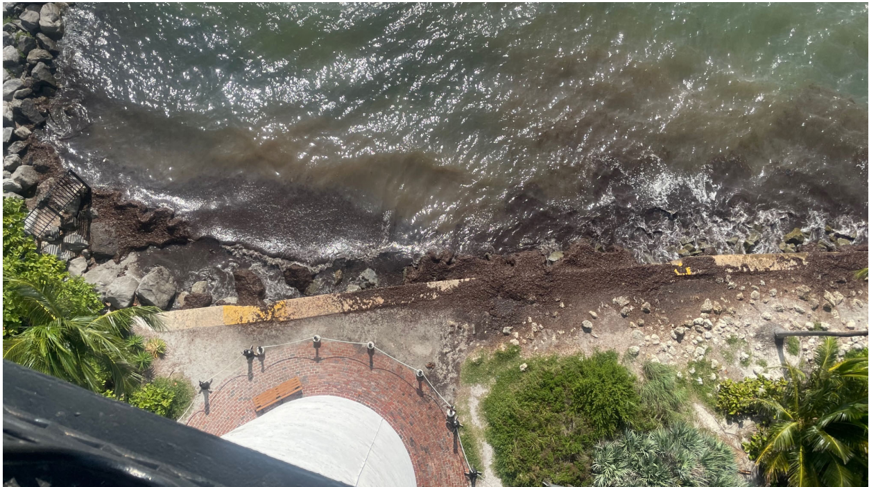
Photo 2-View of King Tides from the Bill Baggs Cape Florida Lighthouse
